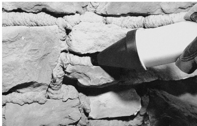
Fig. 21 Lechada con pistola Caulking with the gun
