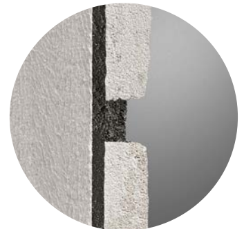
4) spoina cofnięta weld retracted
